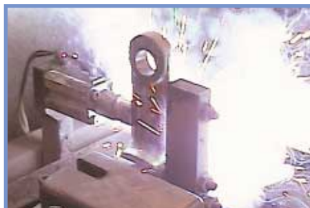
Robotic welding - Automatic welding produces consistent high strength and crack free welding between link and chain flight.
